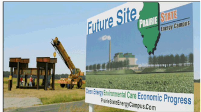
Construction initiated on 1,600 MW Prairie State Energy Campus
